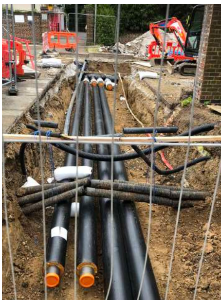
1,200 meters of prefabricated pipework was installed underground between buildings and the Energy Centre
