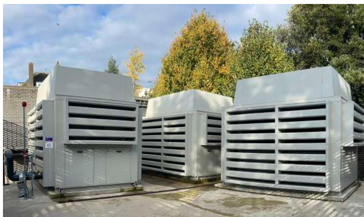
3 x 250kw air source heat pumps with acoustic packs
