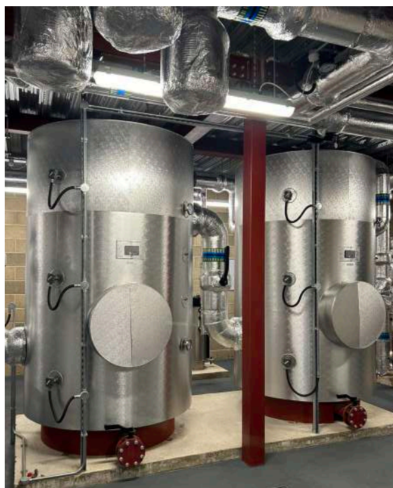
2 x 4,000 ltr buffer vessels that provide thermal storage on the ambient loop
