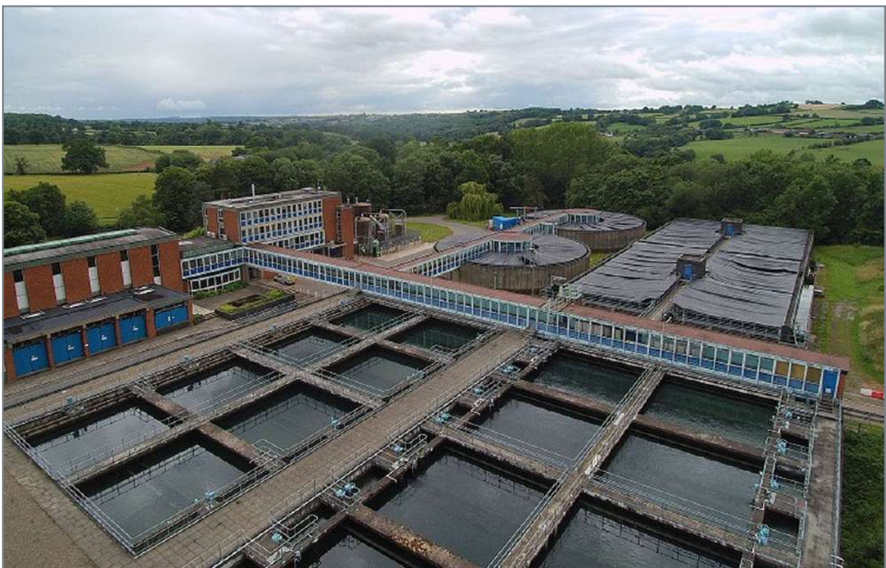
Hampton Loade – South Staff Water Treatment Works
