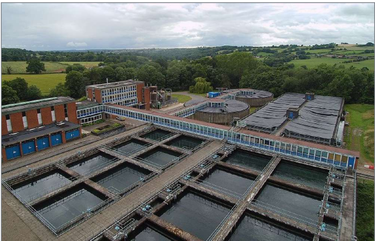
Hampton Loade – South Staff Water Treatment Works
