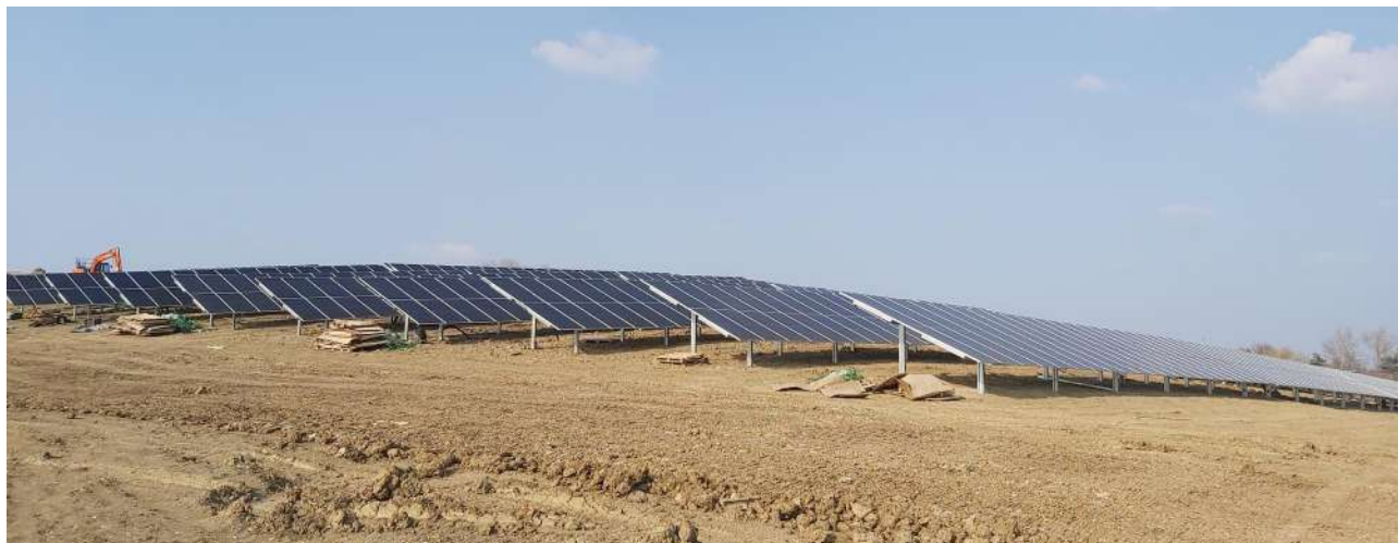
PV panels installation
