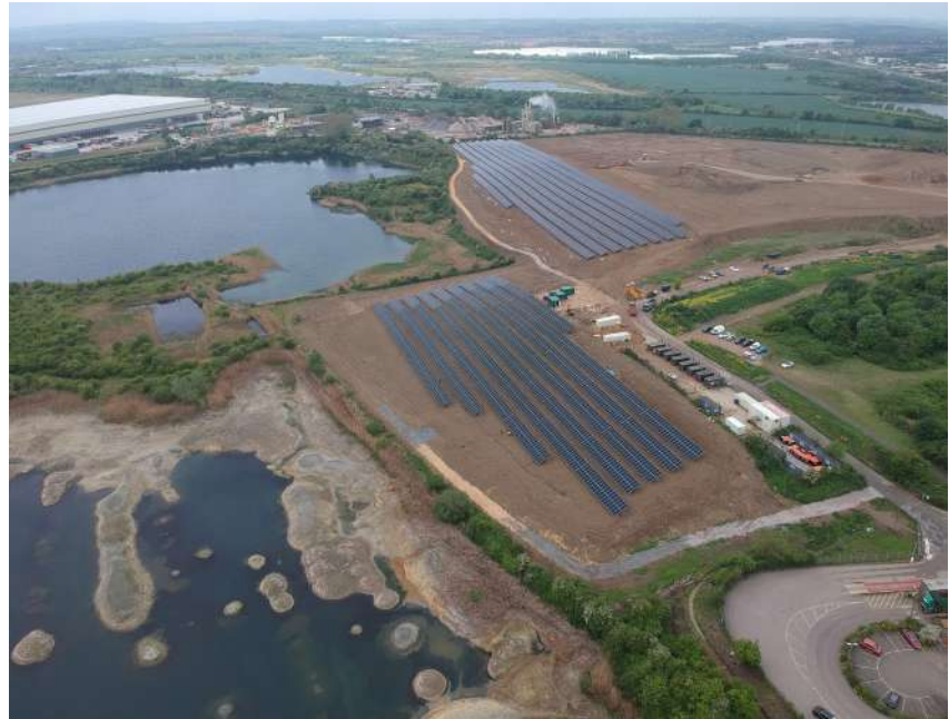
Bedford's Green Energy Innovation Park
