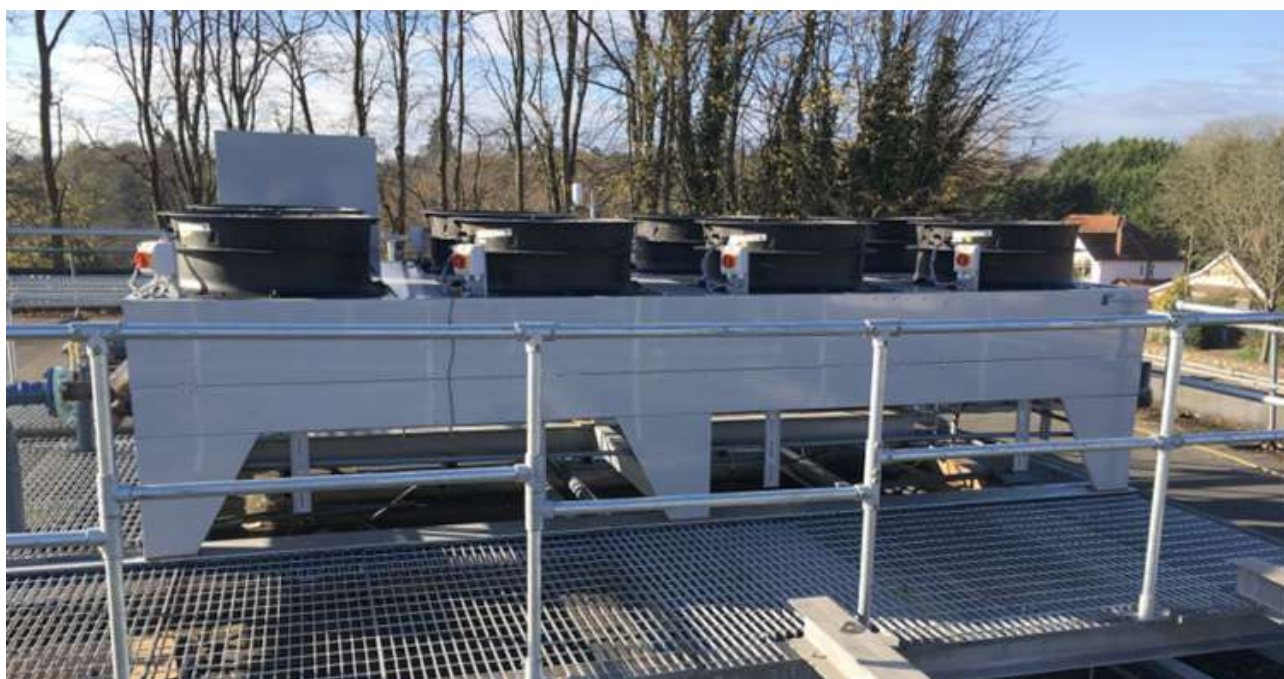
Figure 2 – Roof mounted dry-air coolers
