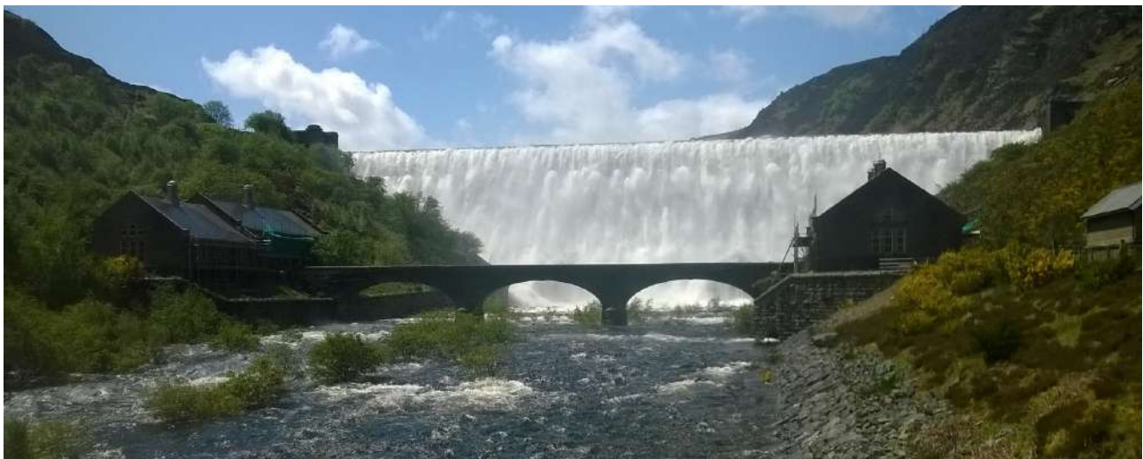
Caban Coch Dam in high spill
