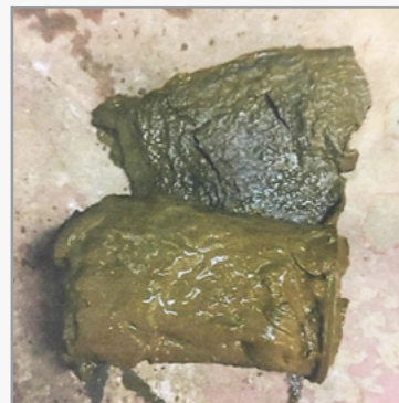
Biofilm removed on an X-POT filter. Biofilm is a greater thermal insulator vs magnetite and scale.
