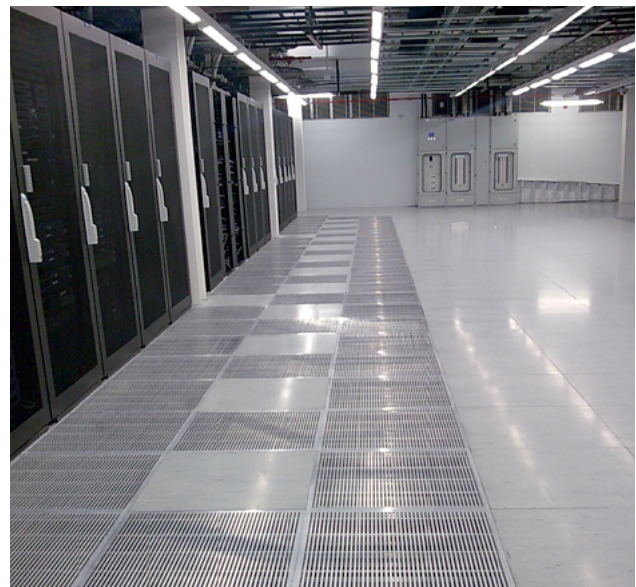
Redundant air terminal grilles contributing nicely to the electricity bill
